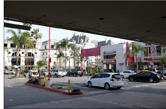
2C. EXISTING STRUCTURE, LOOKING EAST
